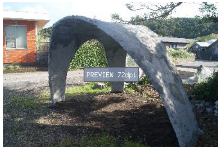
Figure 1. Bamboo reinforced concrete shell.
