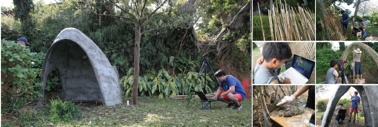
Figure3:Bamboo Concrete Shell 2017 and Construction process
